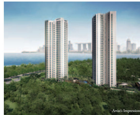
The Meyerise (under construction) • Meyer Road • 239 units Expected Date of Vacant Possession: No later than 1 Oct 2016
